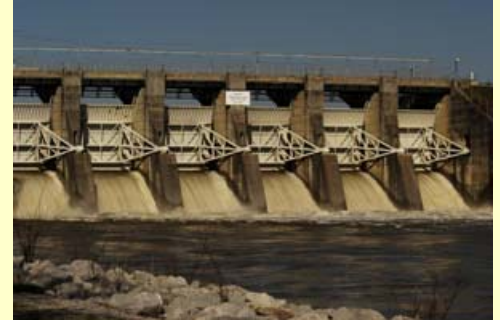
Logan Martin Dam on the Coosa River.
