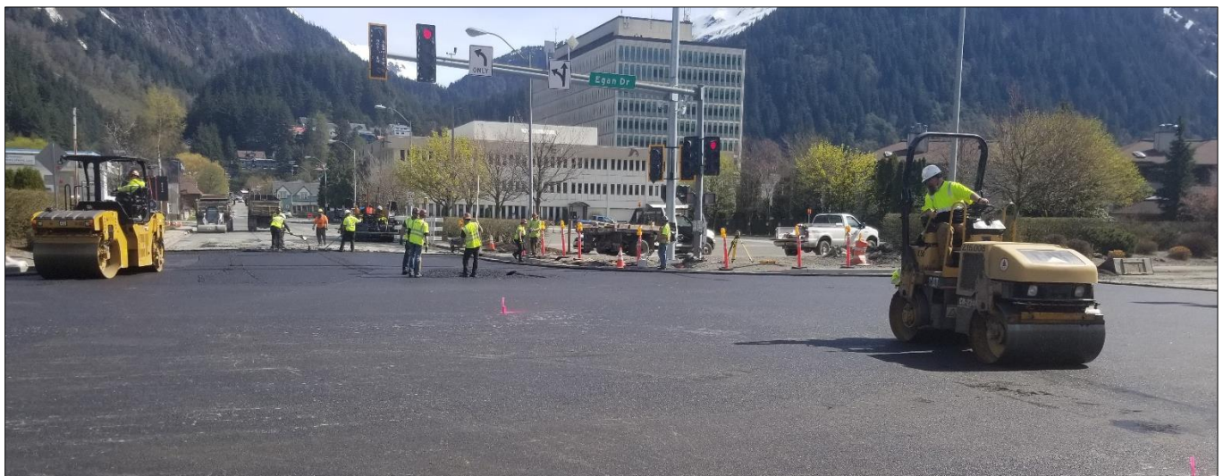
Breakdown and finish rolling the 1 st lift of Superpave HMA at the intersection of Egan Drive and 10 th Street.
