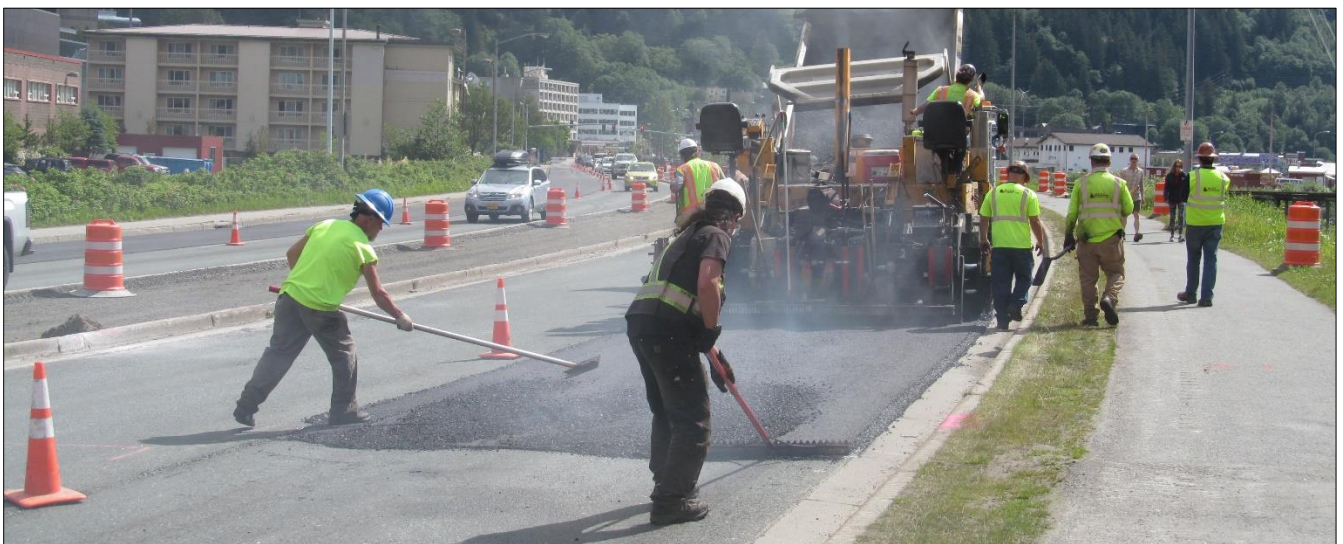
The existing pavement was in such poor condition that some sections scheduled for work in 2020 had to be overlaid with temporary HMA during the 2019 season just to get them through the winter.
