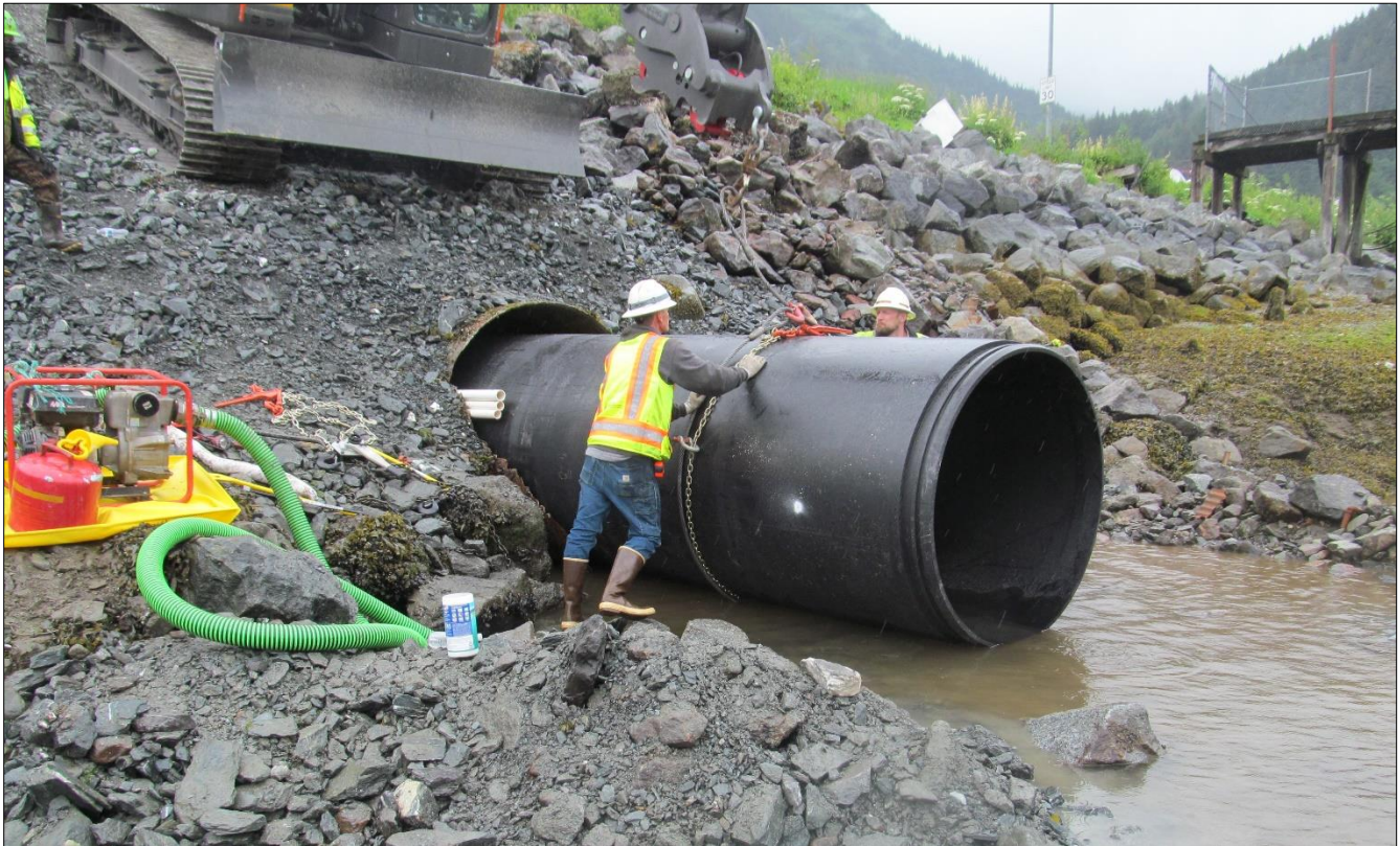
Installing one section of the 140- foot 72" diameter HDPE liner at low tide. Annular spaces were filled with grout.
