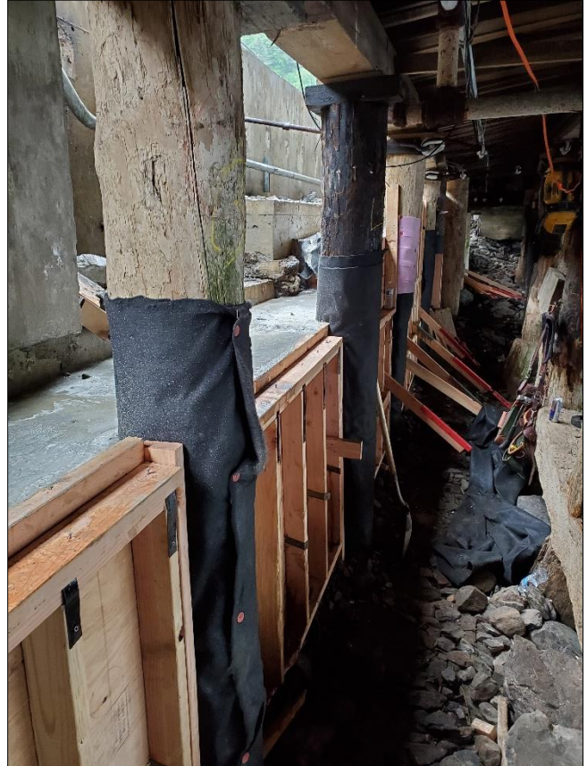
Right: CLSM pour to fill scour voids below footing of existing concrete retaining wall.
