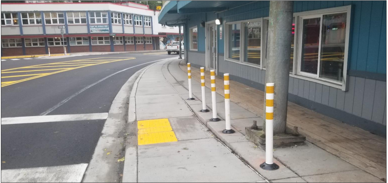
Foreground: Widened sidewalk and ADA-compliant curb ramp in front of Merchant's Wharf. Background: Unsignalized mid-block crossing removed from Seward Avenue intersection.
