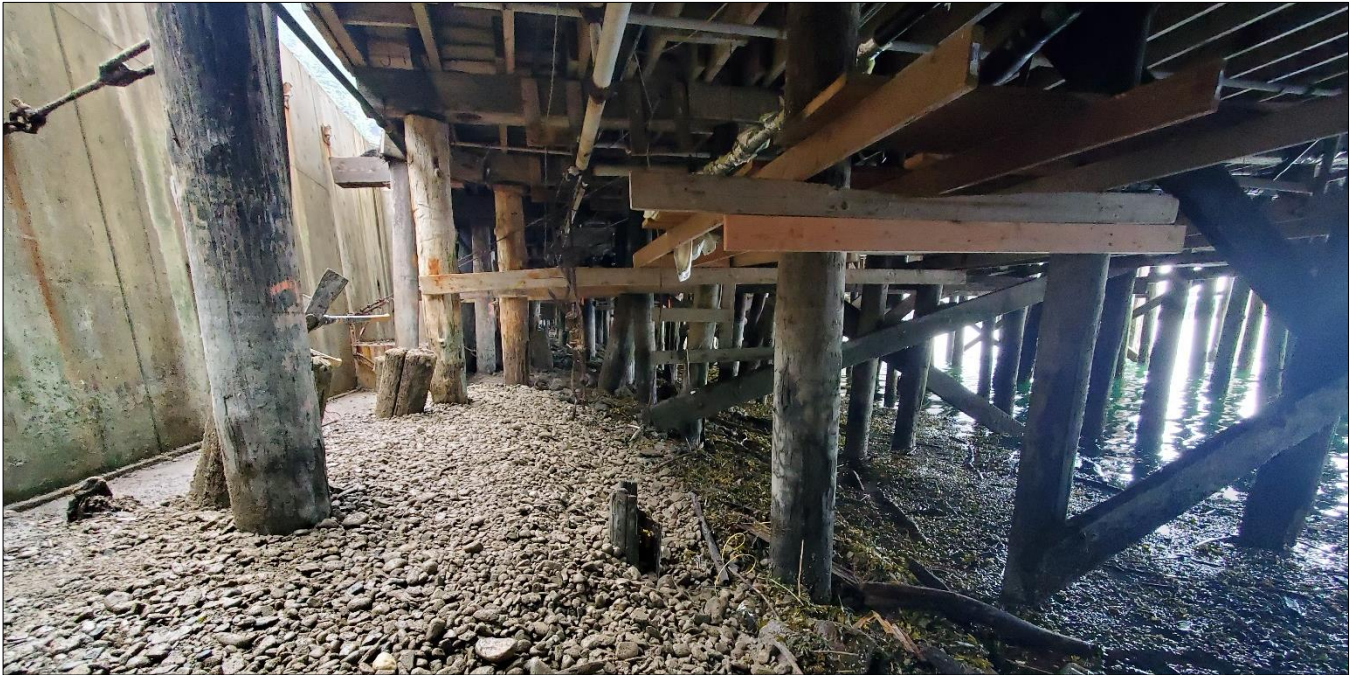
The 'beach' below Merchant's Wharf; existing concrete retaining wall and Main Street intersection at left.
