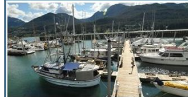
Aurora Harbor Rebuild, Juneau
