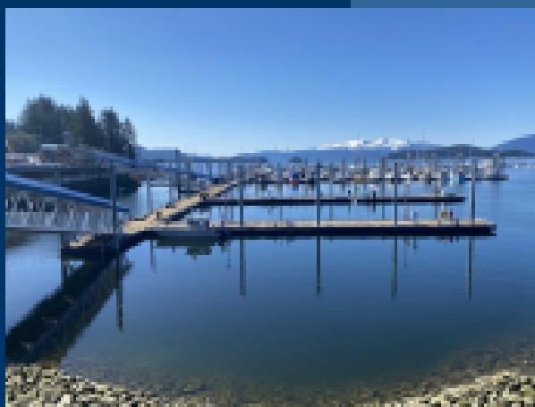
Statter Harbor Improvements
