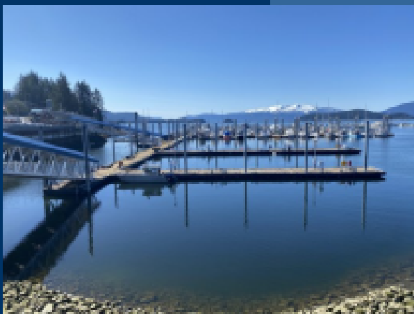
Statter Harbor Improvements
