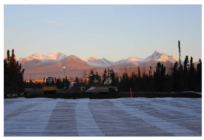
Municipality of Anchorage, 100<sup>th</sup> Ave. Extension, Phase IIA, Minnesota Drive to C Street that was bid and built by Granite in 2016 (completed in 2017). This phase placed a surcharge on the proposed alignment during the winter of 2016-17 to consolidate the underlying peat. The presentation will provide an overview of the project, followed by some of the lessons learned/observed while constructing the project.
