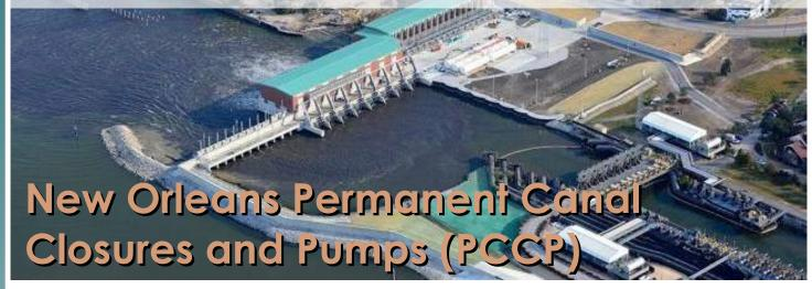
There are three main drainage outfall canals in the City of New Orleans – 17th Street, Orleans Avenue, and London Avenue. These canals are a critical element of the flood control system, serving as drainage conduits for much of the city. This project provides a long-term solution for reducing risk from a 100-year storm event. The solution blocks Lake Pontchartrain surges, which can have wave heights of almost 14 feet, from entering the canals with 18-foot high barrier
