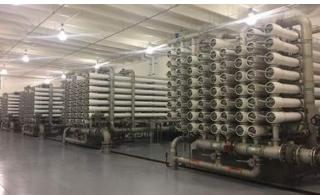
Rob David, SUA operator, conducted the tour of the 35 MGD plant which includes 2.5MGD low pressure reverse osmosis (LPRO) and 32.5MGD nanofiltration (NF). Water for NF is pulled from 36 shallow wells (~175 feet deep) and water for LPRO from additional deep Floridan aquifer wells. LPRO concentrate is injected into the boulder zone while NF concentrate travels 7 miles to the wastewater treatment plant where it is reclaimed.
