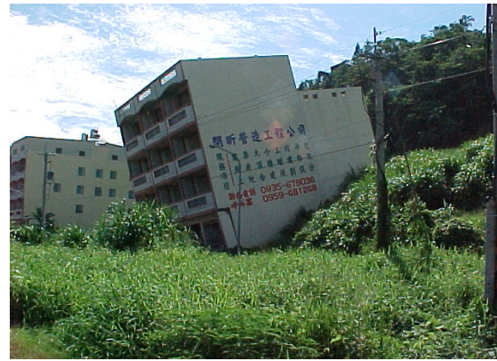
Figure 8 Reinforced Concrete Building Tilted by about 4.5 m of Reverse Fault Displacement without Collapsing
