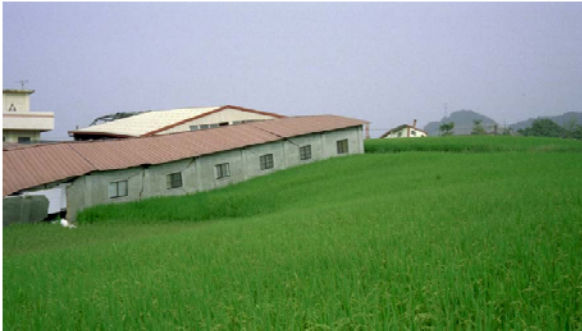
Figure 6 Ground Warping Associated with the 1999 Chi-Chi Earthquake (photo by N. Sitar)
