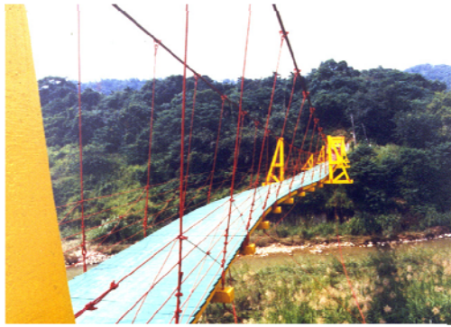
Figure 12 Suspension Walkway Bridge Undergoing Relative Movement of its Abutments due to Fault Movement (photo by C. Roblee)
