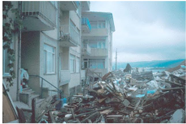
**Figure 7** Apartment house shown on right side of photo, which collapsed due to surface rupture. Fault passes across the middle of the photo between the two standing apartment houses; the far apartment house has been offset about 3 m from its original alignment with the near apartment house (Photo by F. A. Swan from Lettis et al. 2000).
