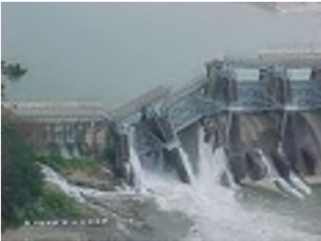
**Figure 15** View to the east of surface fault rupture through Shihkang Dam (Photo by J.D. Bray).
