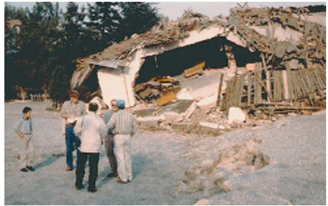
**Figure 11** Fault rupture destroyed a primary school building in Kullar (Photo by L.S. Cluff; from Lettis et al. 2000).
