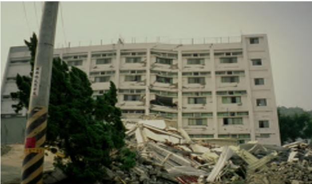
**Figure 19** The primary trace of the Chelungpu fault passed beneath this apartment building in Wu Feng, producing about 2 m of vertical displacement through the building (Photo by K. Kelson).
