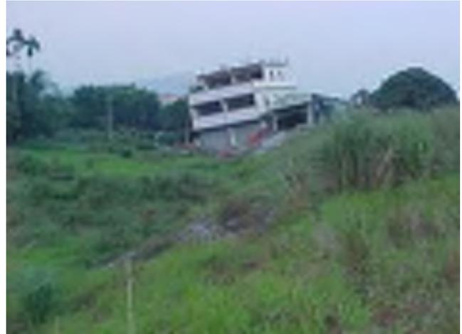
**Figure 20** North-facing subsidiary fault in hanging-wall block and local ground deformation damages this house and warehouse. This site is located southeast of Shihkang Dam and south of the primary fault ruptures running along the Tachia River in this area (Photo by J. Bray).
