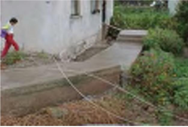
**Figure 13** Well-built 2-story house in Arifiye is not damaged although the primary surface fault scarp passed beneath it with over 3 m of right-lateral displacement. In response to the underlying fault movement, the stairs leading to the house have been offset relative to the house (Photo by J.D. Bray).
