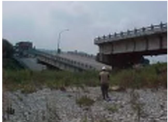
**Figure 17** Collapse of bridge directly east of Shihkang Dam due to tectonic compression (Photo by J.D. Bray).
