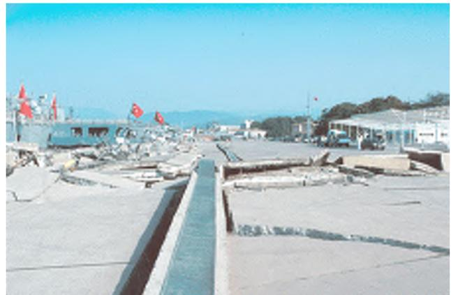
**Figure 9** Fault offset of about 2 m heavily damaged this dock at the Gölcük Naval Base, which was fixed to the ground with piling (Photo by F.A. Swan; from Lettis et al. 2000).
