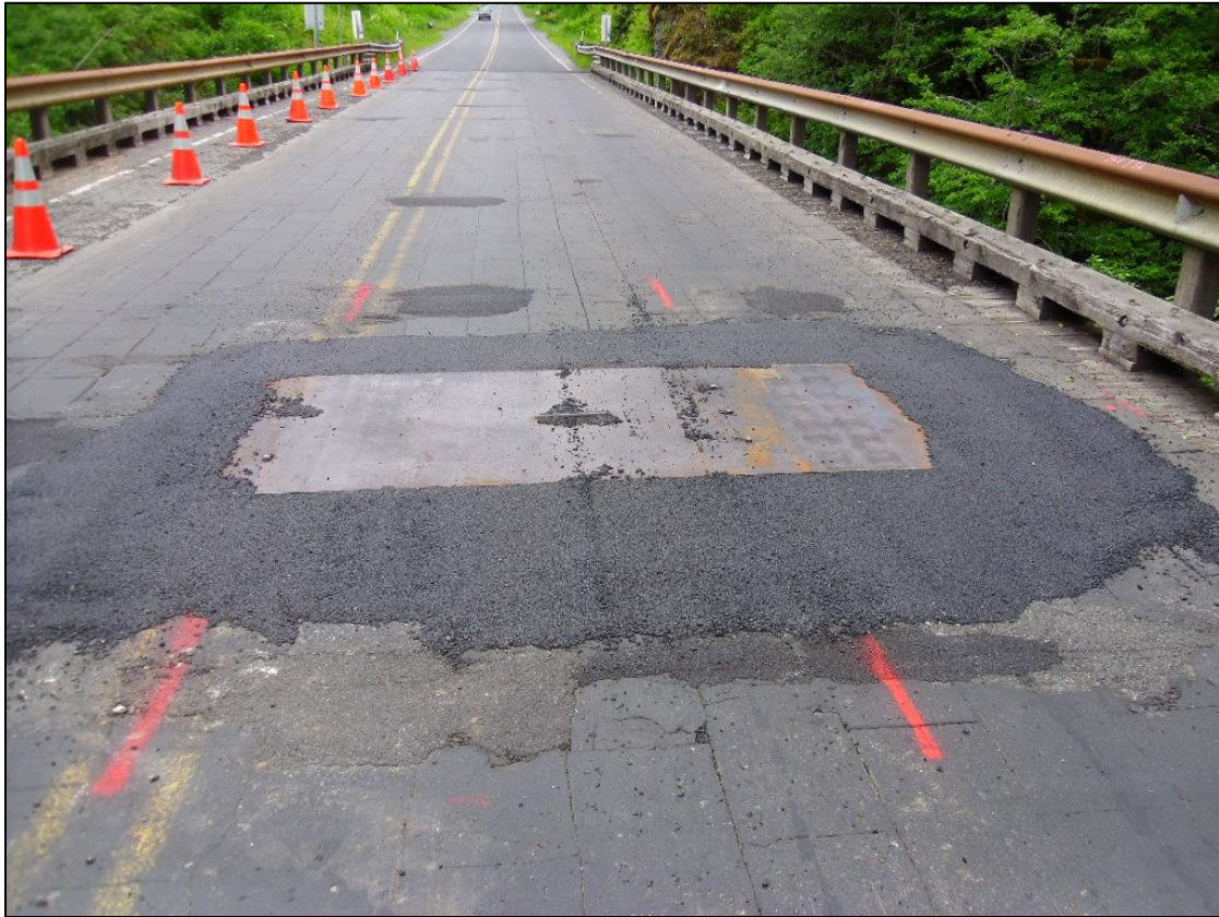
The Old First Waterfall Creek Bridge with Closed Shoulder and Deck Repairs
