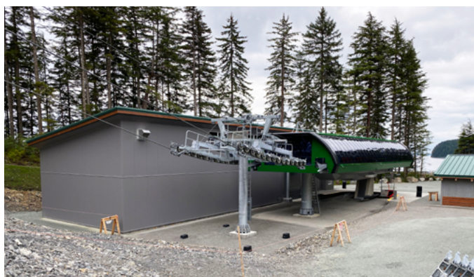
TRANSPORTER Gondola storage building
