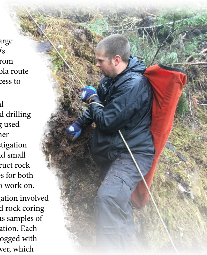
PND Principal Engineer Sean Sjostedt, P.E., using a static line during the geotechnical investigation
