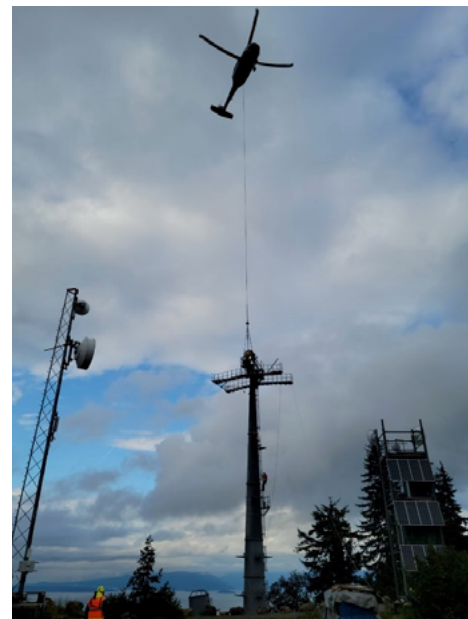
Helicopter transport of tower component during construction
