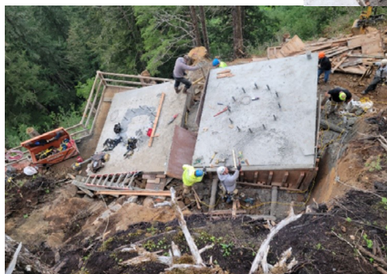
Construction of tower foundation being performed on steep terrain using benches
