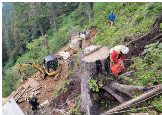
Construction of tower foundation being performed on steep terrain using benches
