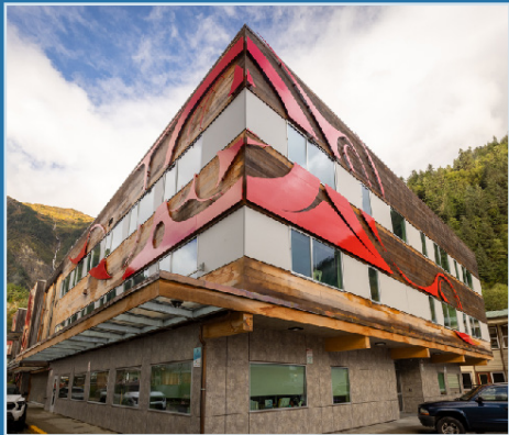
SHI Indigenous Science Building Photo by SHI
