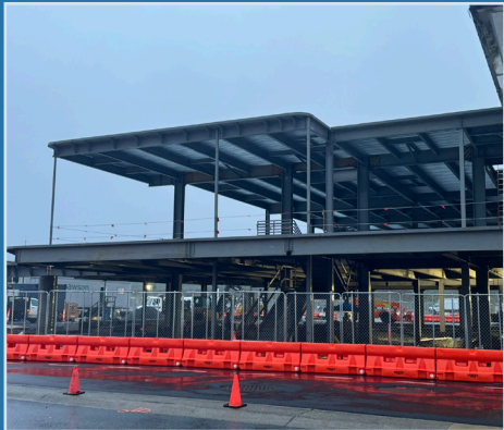
Ketchikan Airport Addition
