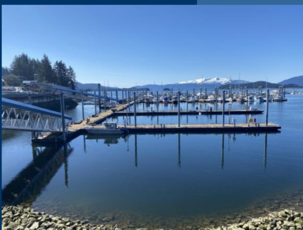
Statter Harbor Improvements
