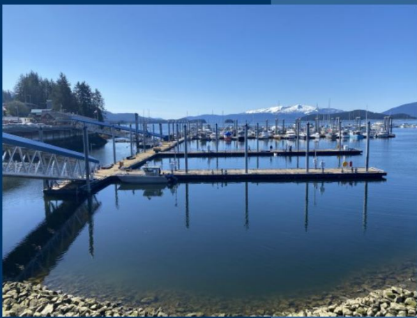
Statter Harbor Improvements
