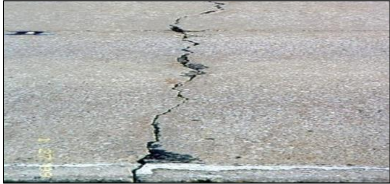
Thermal Stress Cracking
