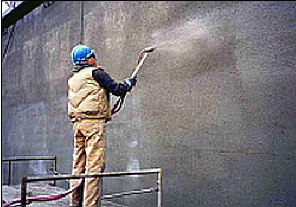
Crystalline Slurry - Spray Applied
