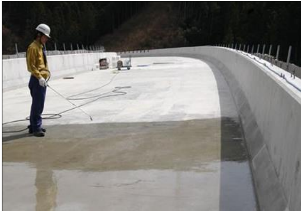
Modified Silica Gel – Spray Application
