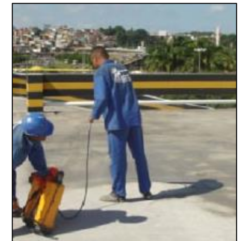
Modified Silica Gel – Spray Applications
