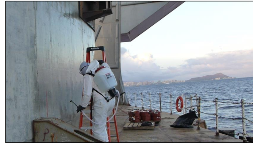
Modified Silica Gel – Spray Applications
