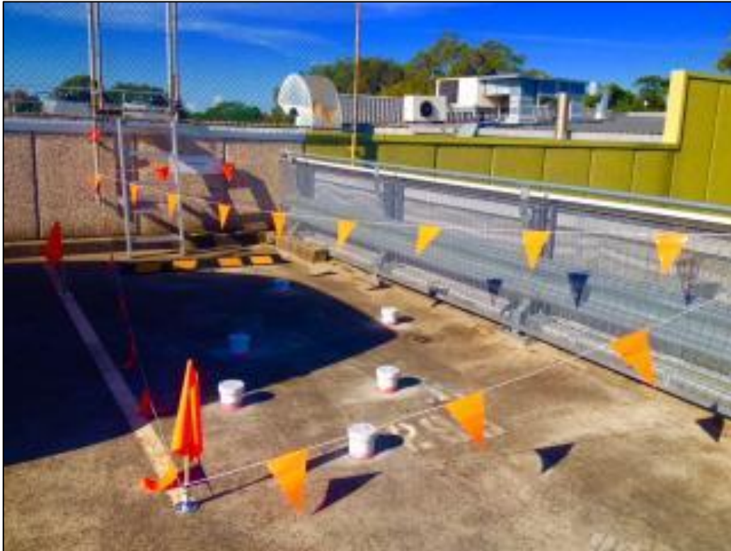
2017 Water Test being conducted (6 locations – 3 over cracks & 3 over solid surface)
