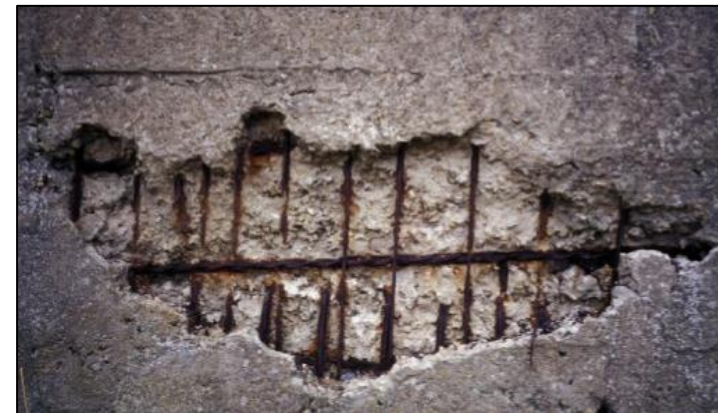
Spalling caused by Corrosion of the Steel Reinforcement
