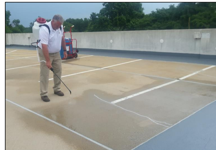
Modified Silica Gel – Spray Applications
