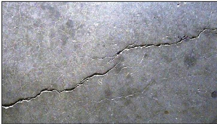
Shrinkage Cracking
