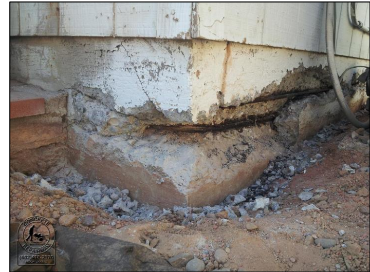
Temperature & Moisture Deterioration
