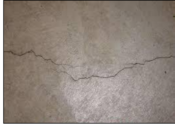
Stress Cracking
