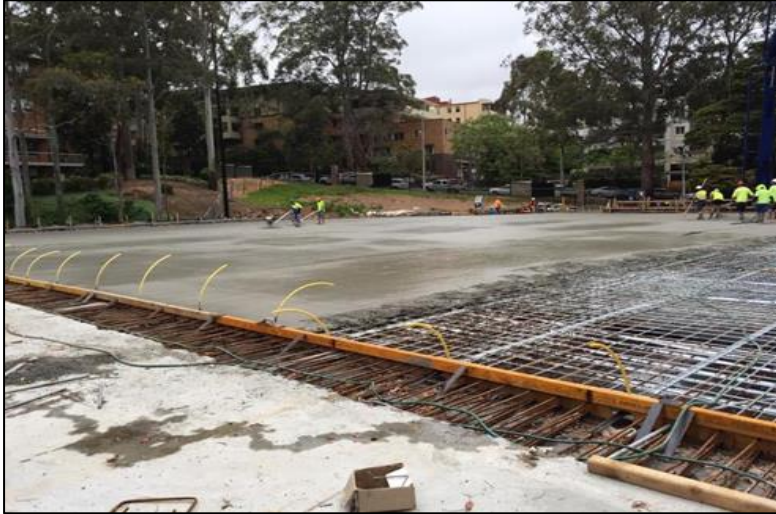
Construction of Concrete Slab
