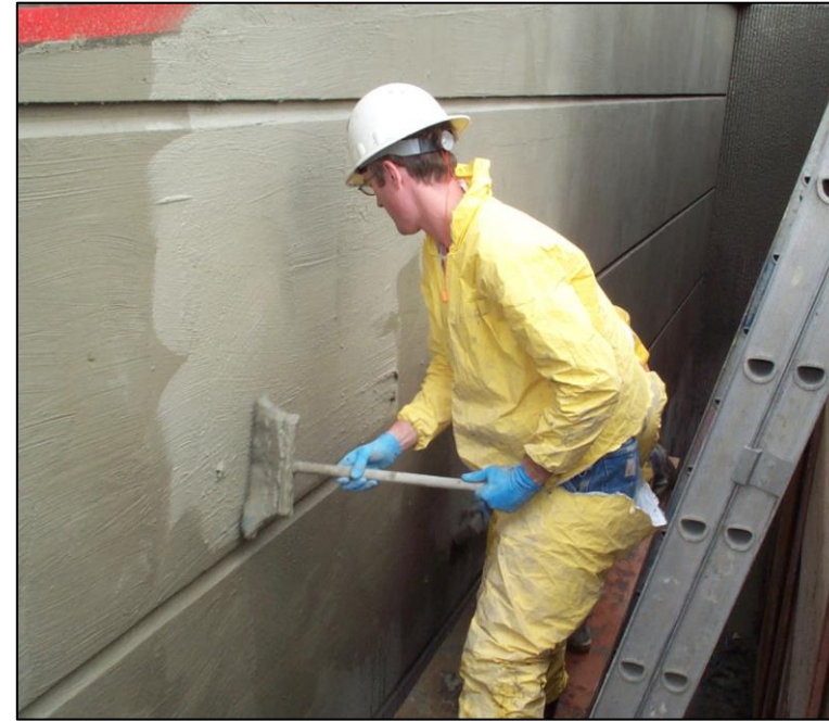
Crystalline Slurry – Brush Applied
