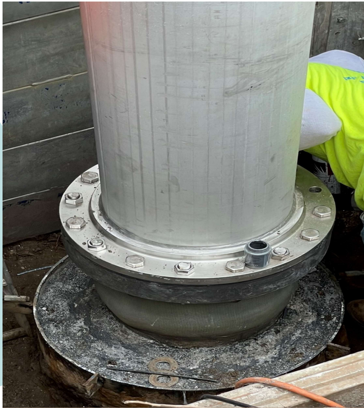
New well casing
