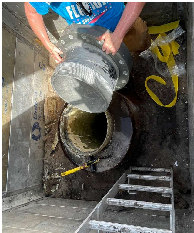
FRP Casing Repair
