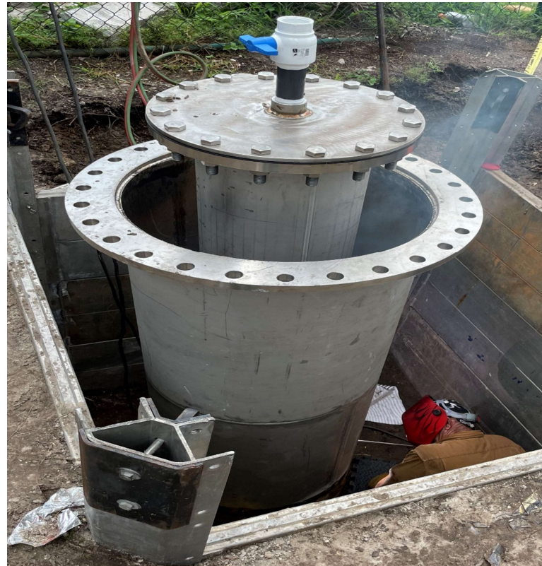
New surface casing
