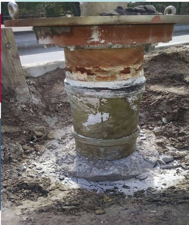
FRP Casing Repair
