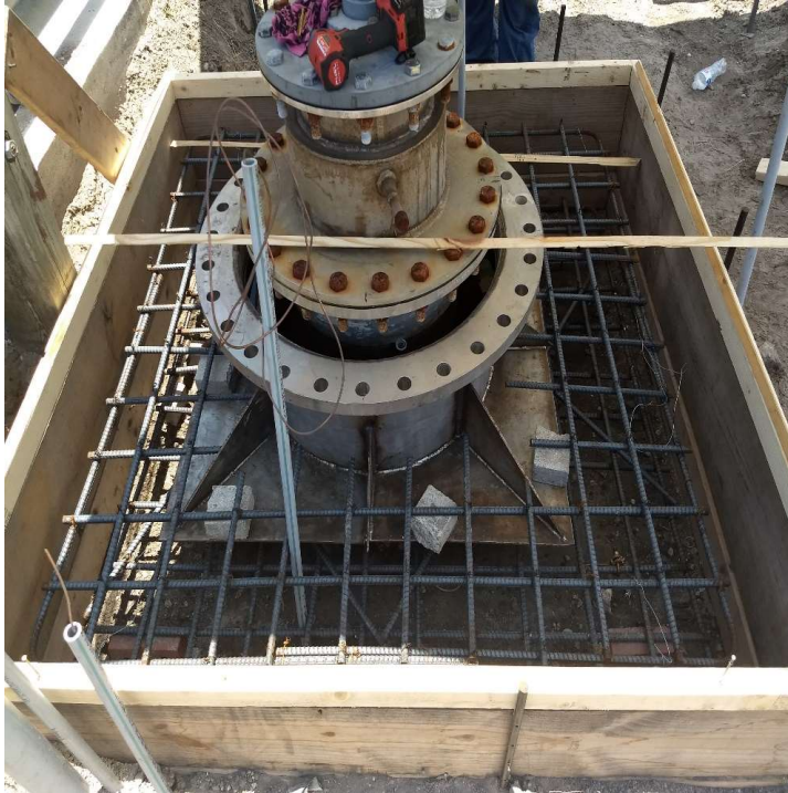
Well pad reinforcement with gusset plate to surface casing
