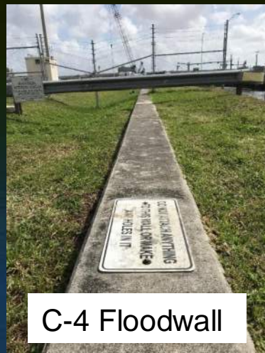
Raised Canal Banks (conveyance)
