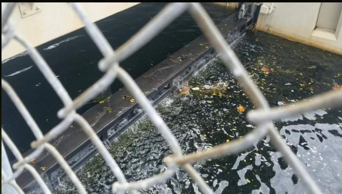
October 2019: Gates closed, high tide water reverse flowing over the top
