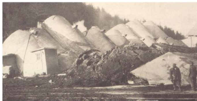
Figure 5-2: Bearing Capacity Failure of Silo Foundation (Vesic, 1975, from Tschebotarioff, 1951)
