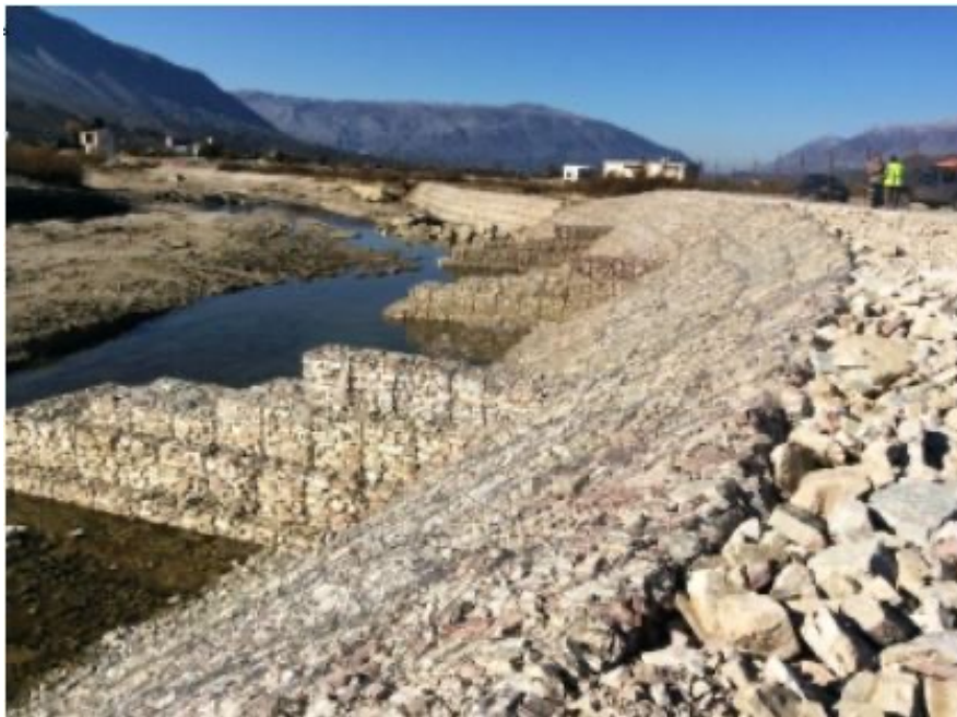
Figure 6.3 Gabion boxes (wire cages containing stones) strengthen the banks (Source: Knapp et al, 1989)
